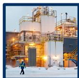
Power to Gas Bécancour 20 MW Electrolyzer PEM Technology
